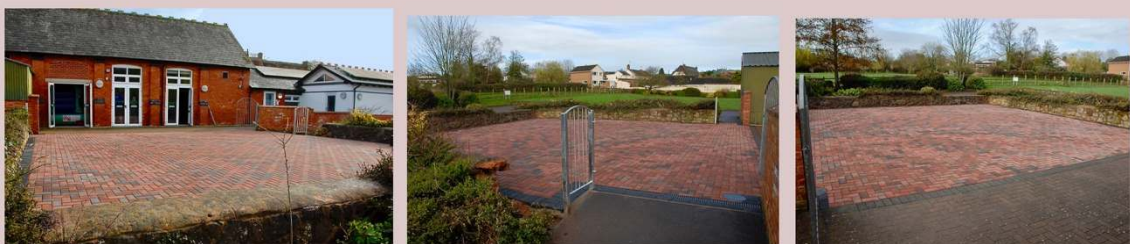
The new Terrace area at TMH is close to completion
